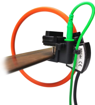
Copper row bracket installation
